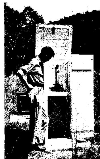
FIG. 4. GROUND-WATER WELLS FOR DETERMINING ELEVATIONS OF THE WATER TABLE
