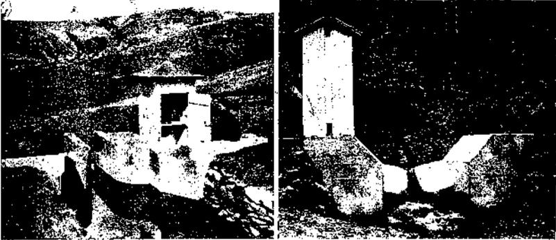
FIG. 2. A 2-FT SAN DIMAS FLUME IN THE COPPER BASIN EXPERIMENTAL AREA, TENNESSEE
