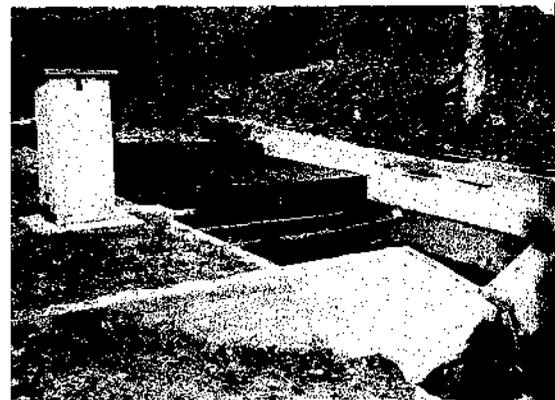
FIG. 1. A 120-DEG V-NOTCH WEIR INSTALLATION WITH SILTING BASIN, PONDING BASIN, AND BY-PASS
